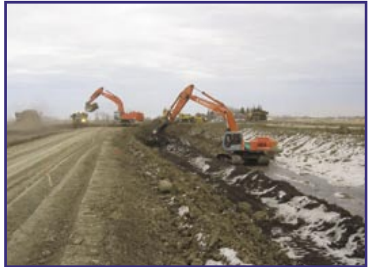
Work underway on Secondary A canal. WID photo
