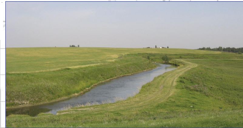
This is a section of A Canal prior to rehabilitation. WID photo
