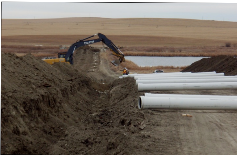
Pipe lays ready to be installed near Redland. -WID Photo
