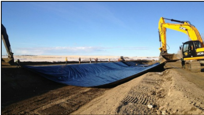
Canal liner install in secondary A canal - WID photo
