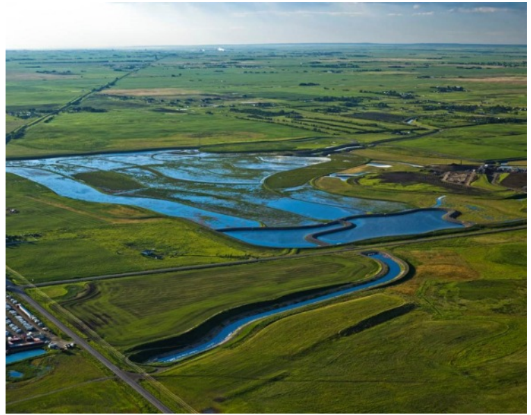
Shepard Wetland in Calgary provides a holding area for storm water during major rainstorms - Ch2M Hill - photo
