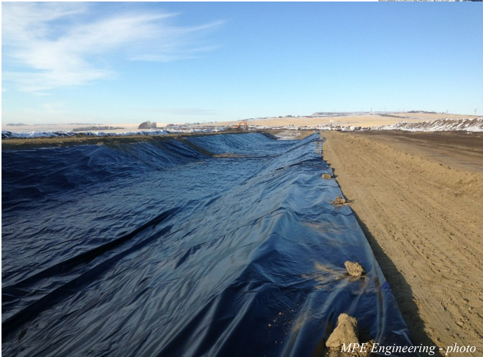
Plastic canal liners significantly decrease loss of water through seepage
