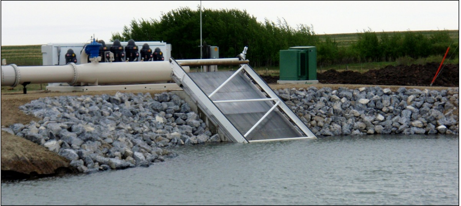
This is the first year in the WID's history that irrigation water is supplied by anything more than gravity. This pump station, installed along the Stoodley pipeline, is capable of providing pressure up to 45psi and 20,000 gallons/minute. - WID photo
