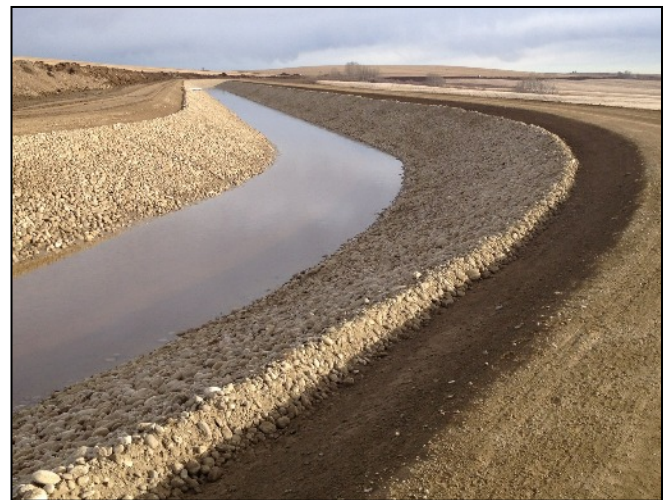
Plastic liner installed in A canal decreases seepage, and gravel armour along the edges reduces erosion. - WID photo
