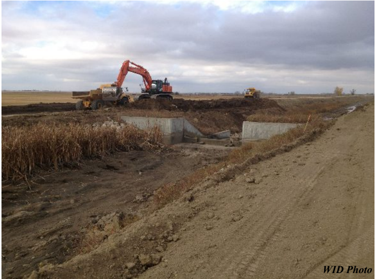
Construction on Secondary C Canal was well under way in the early fall. Lining the canals or converting them to pipeline creates huge water savings.
