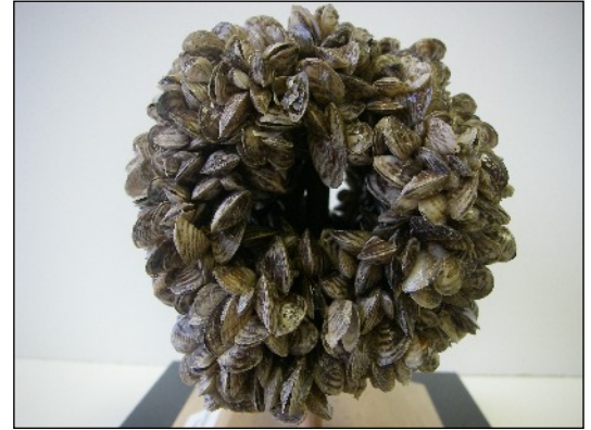
Quagga mussels can take over a pipe like the one above in 6 months or less. Alberta Government, photo
