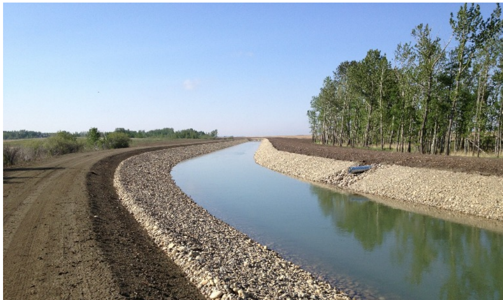
Gravel covered poly liner installed in C Canal decreases seepage - WID photo
