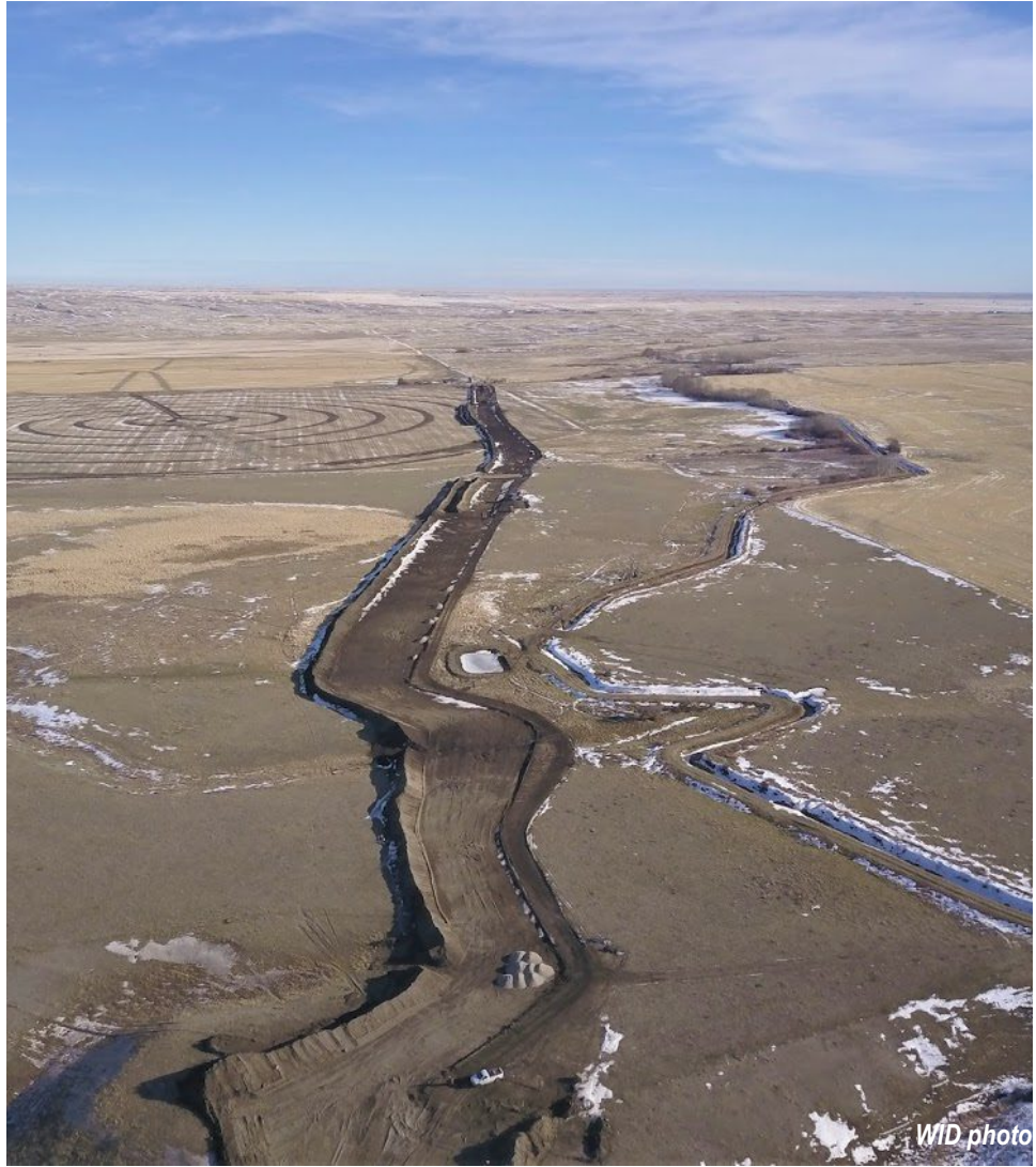
The North Cluny Tailout improvements will eliminate evaporation and percolation losses.
