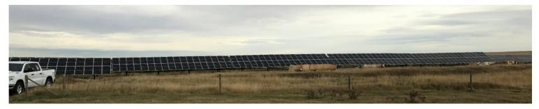
The WID is harnessing the power of the sun to move water through a portion of its system. On October 16<sup>th</sup> the WID commissioned a 500 kW solar generation system at the Stoodley Pump Station. This system is intended to entirely offset the energy usage of the pump station over the course of a year.
