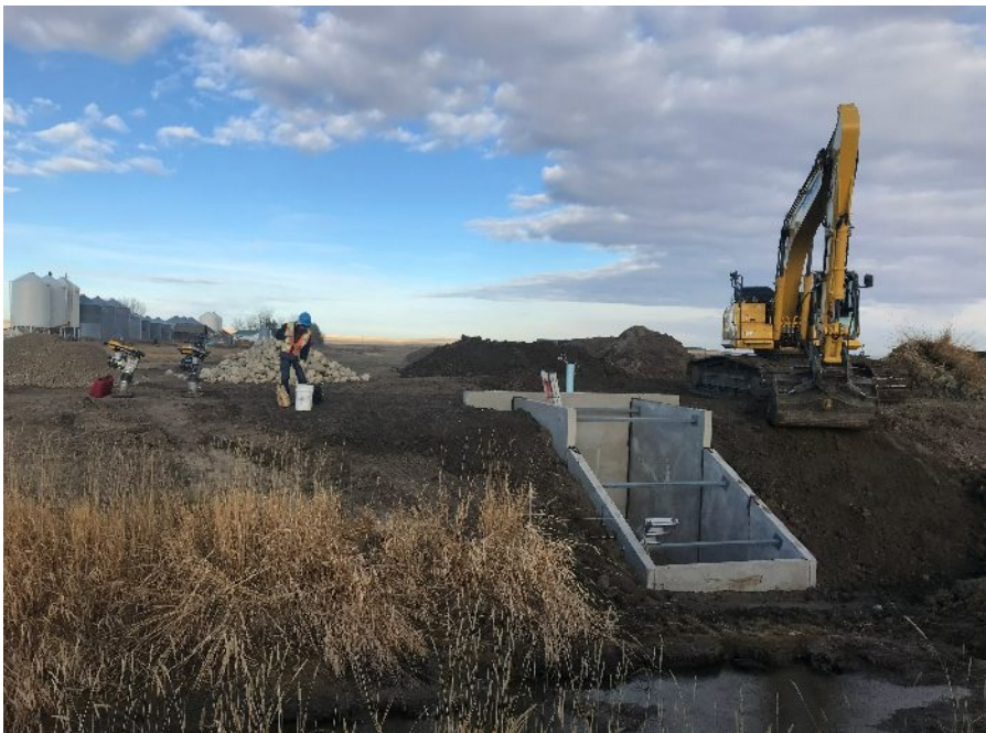
Construction of Hayes Spillway - WID photo
