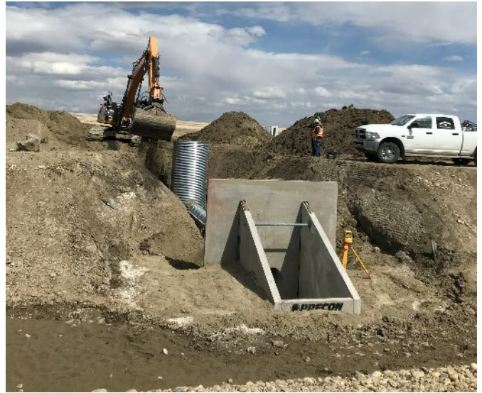
Installation of structure on Standard Canal - WID photo
