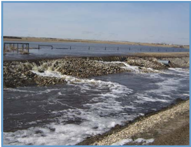
Overland flooding causing bank erosion and armour washing
