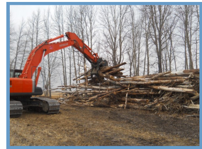
Tree clearing by Carseland
