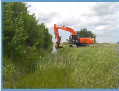
Cattail cutting near Langdon
