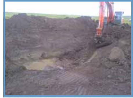
Dugout excavation east of Strathmore
