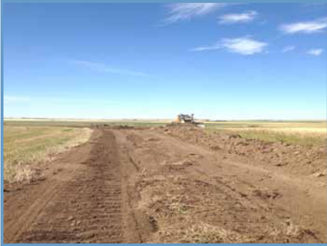
Ditch backfilling near Gleichen
