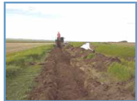
Canal bank repairs NE of Strathmore
