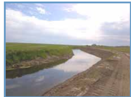
Silt removal and slope protection NE of Strathmore
