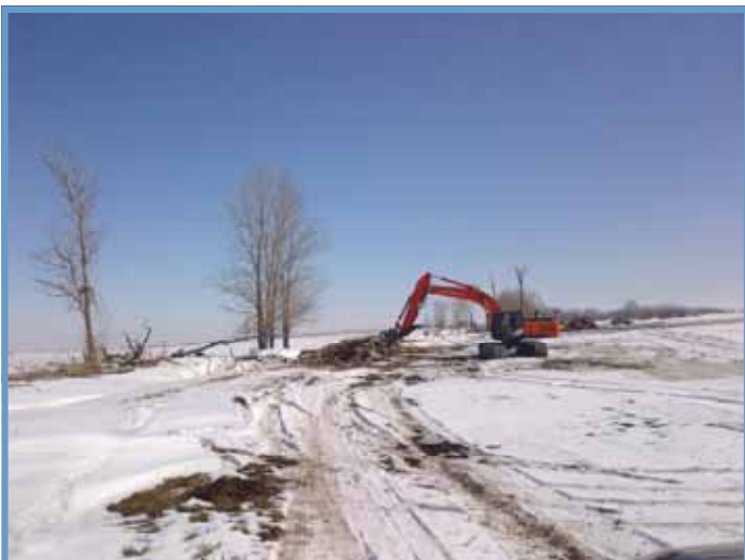
Tree clearing by Carseland
