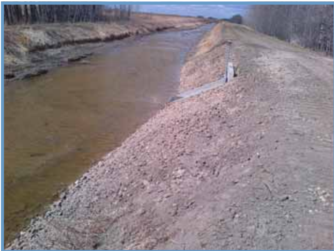
Canal inlet structure near Keoma
