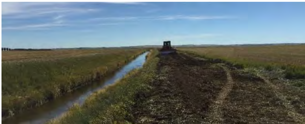
Silt berm levelling east of Strathmore
