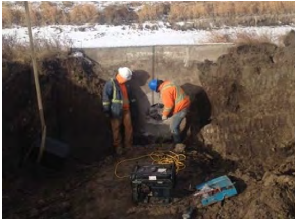
Culvert replacement NE of Strathmore
