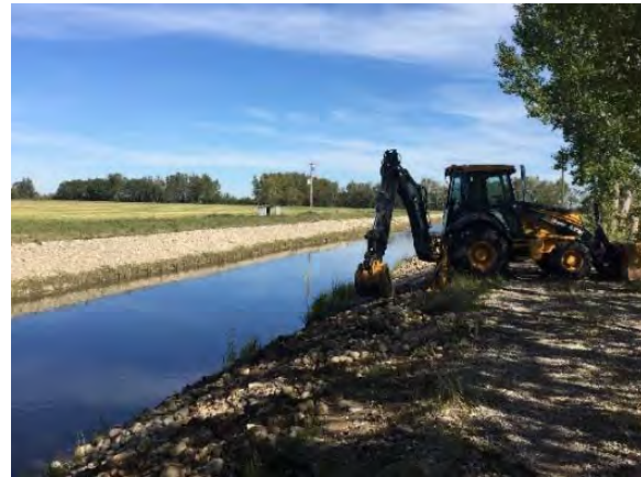
Armour repairs near Strathmore
