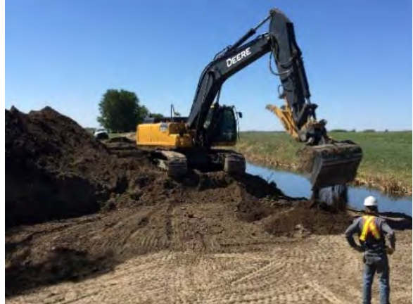
Structure replacement north of Strathmore
