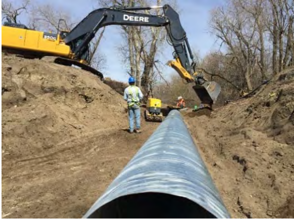
Spillway access crossing NE of Strathmore
