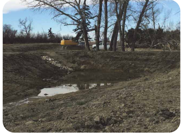
Enhanced stock water dugout and new delivery near Cluny
