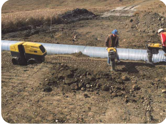
Access crossing replacement near Strathmore
