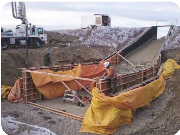
B Canal Structure Repair
