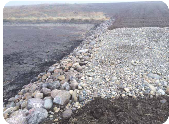
North A Canal Tailout Repair
