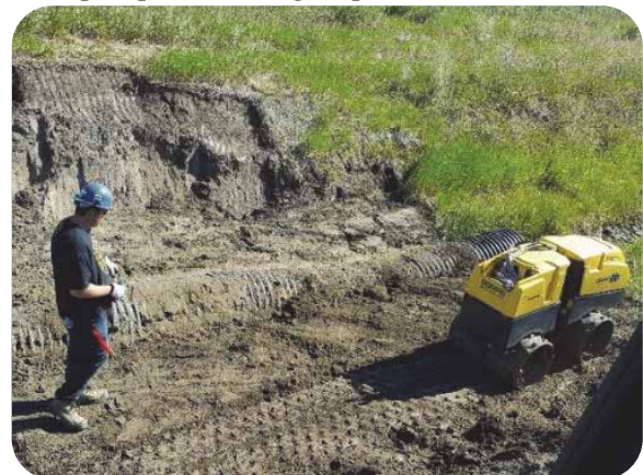
Drop Pipe Crossing Repair near Gleichen
