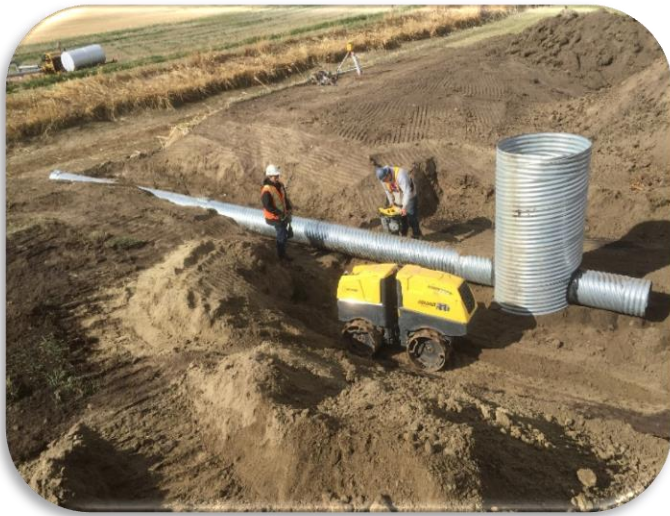
Irrigation Stand Pipe Installation
