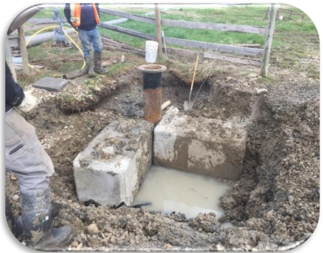
Thrust Block Installation
