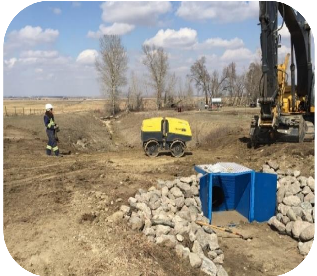
Check Box Installation
