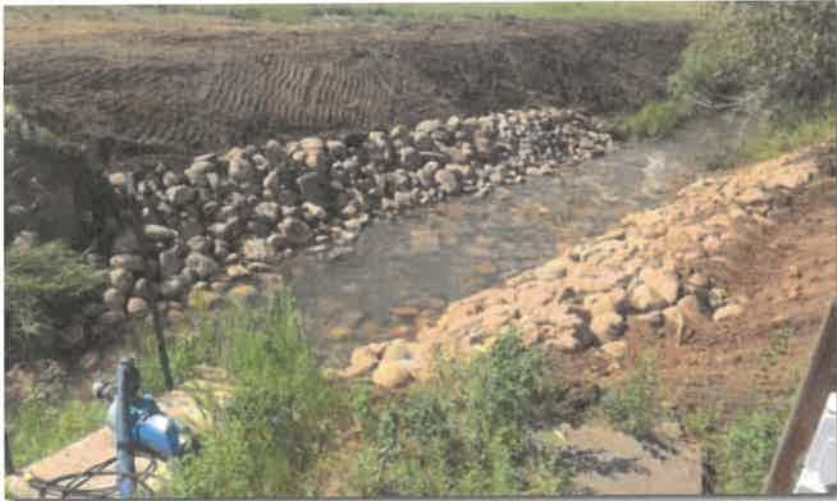
Washed out drop pipe replaced with rip rap
