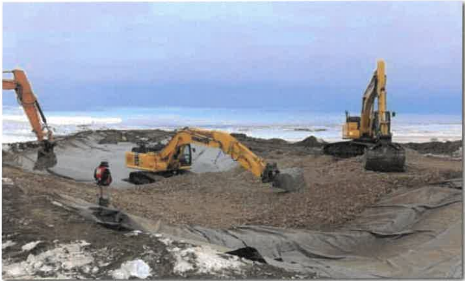
Installation of liner and armoring on Glenrose Canal system
