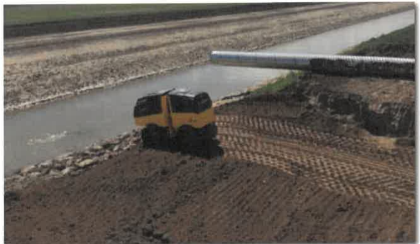
Field drain inlet installation repair
