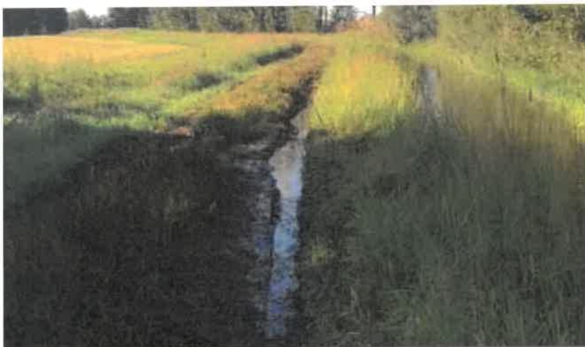
Seepage issues Cairnhill North Ditch
