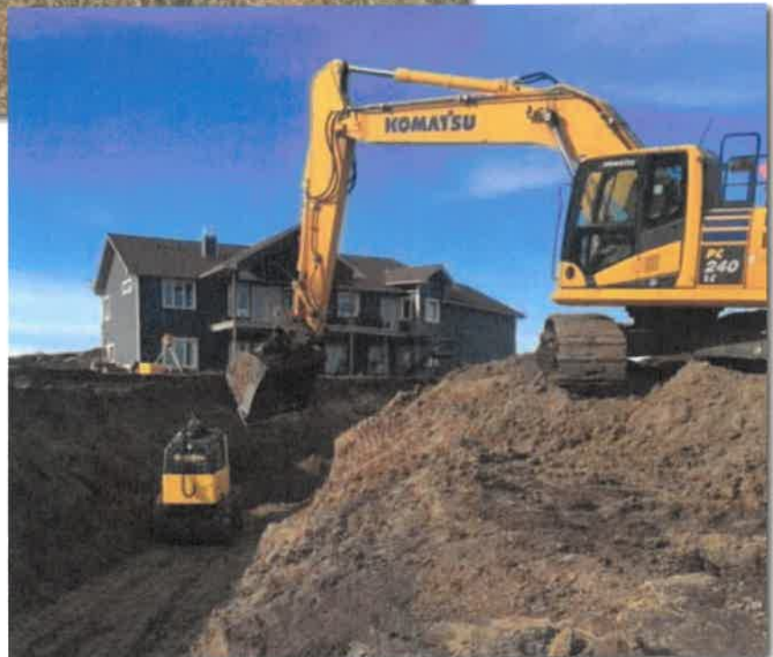
Yard water pipeline installation near Highway 21
