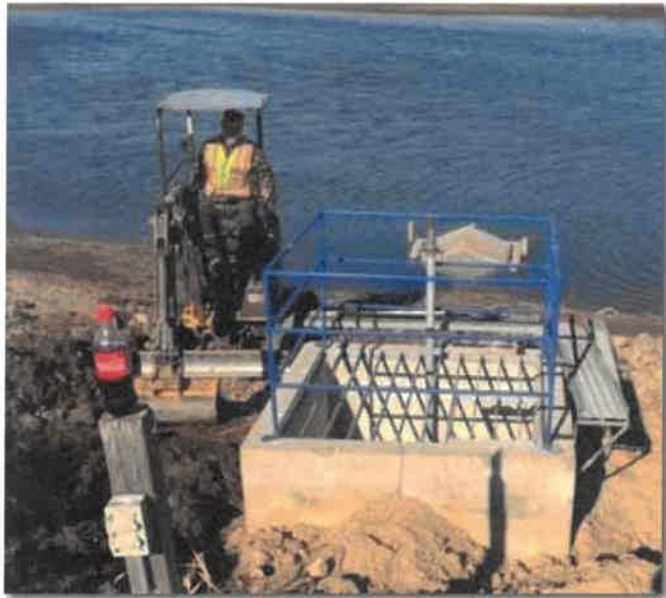
Dalemead Reservoir vault repair
