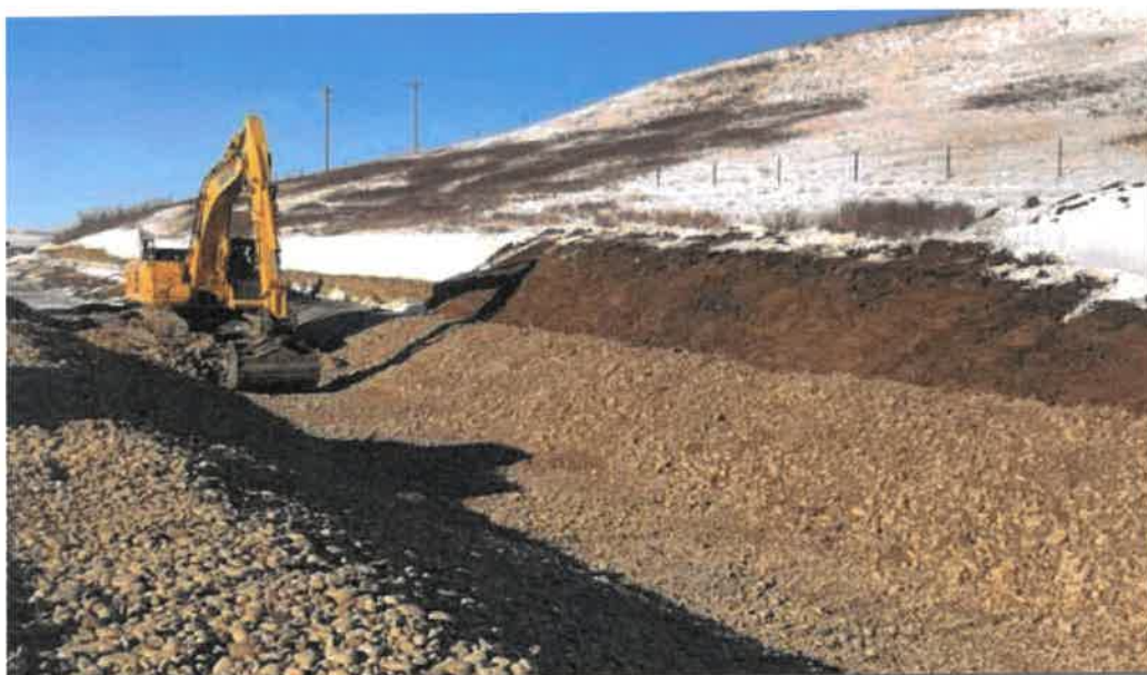
Finished armor placement on poly liner
