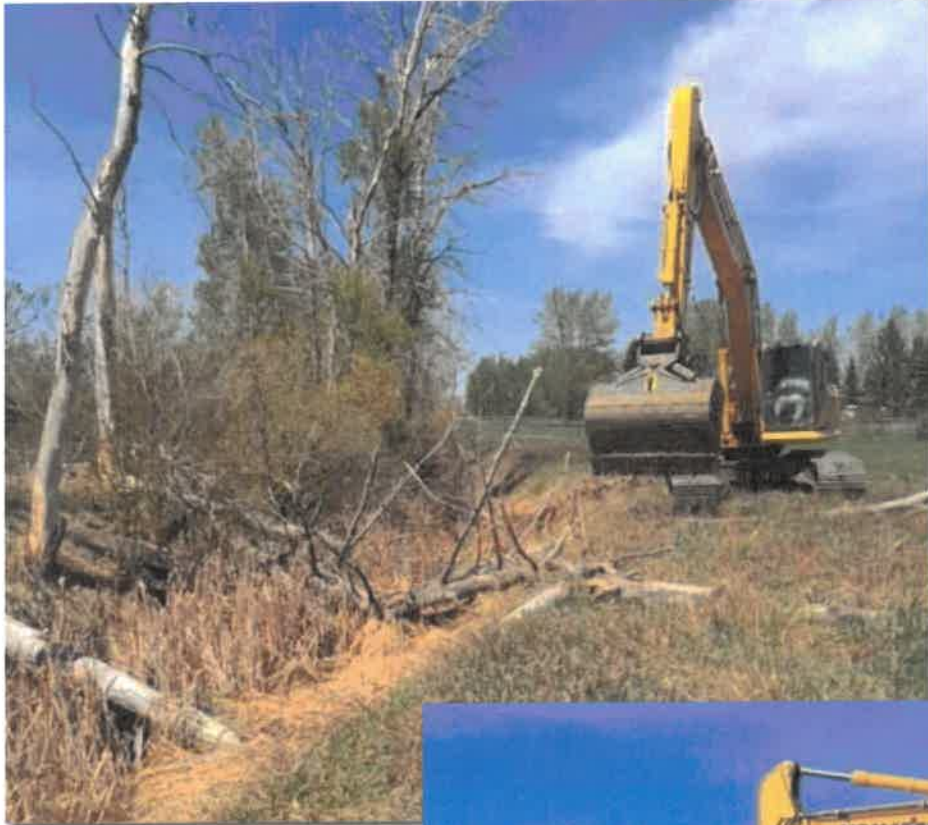
Ditch cleaning Carseland Area
