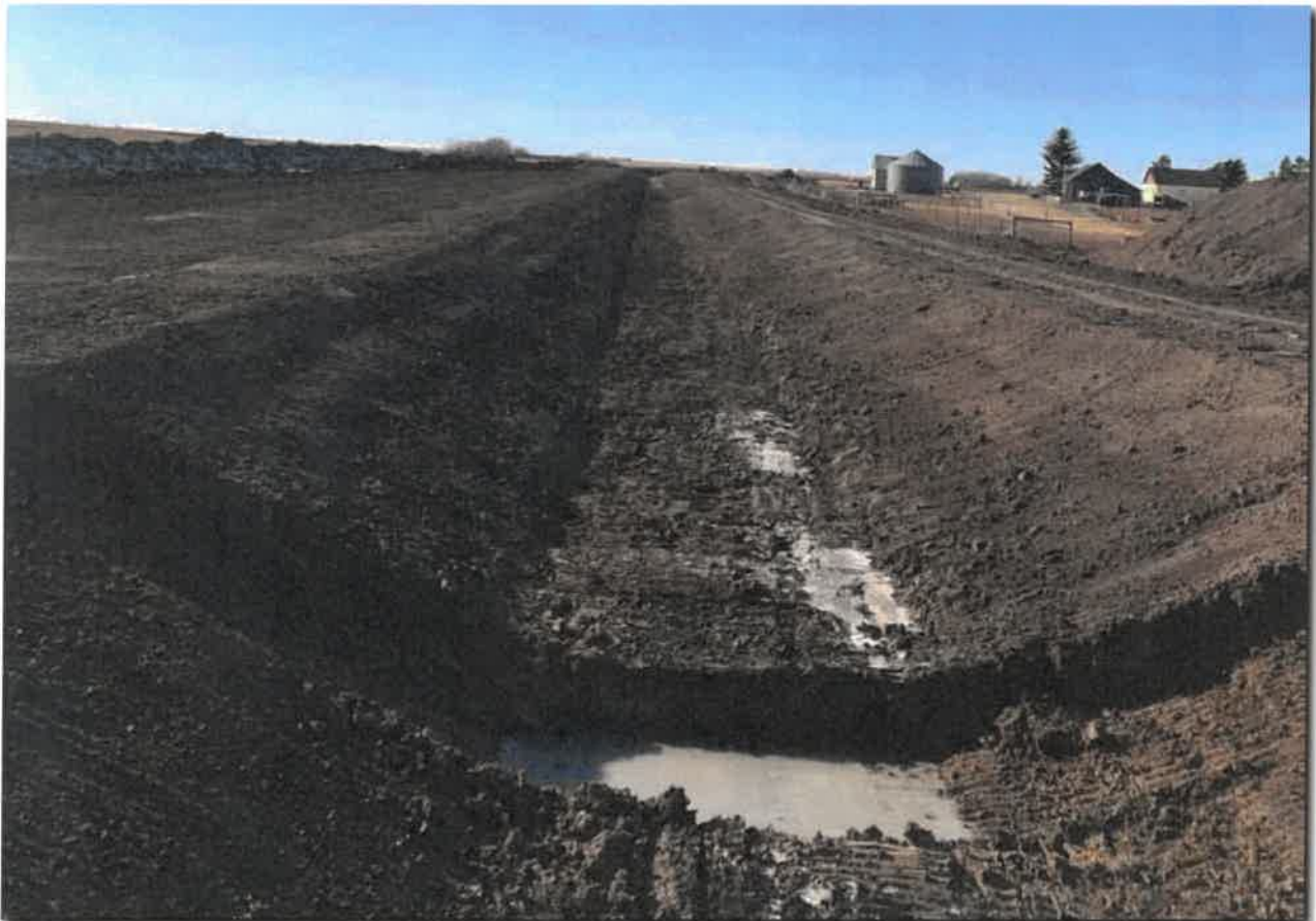
Canal sub-grade prepared for liner installation
