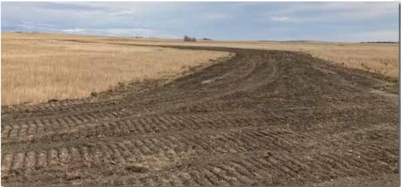
After decommissioning of legacy infrastructure
