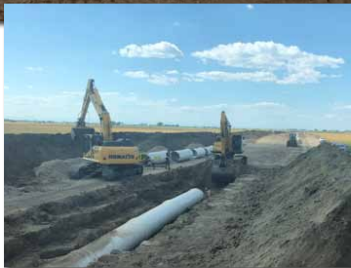
Mainline installation and backfill
