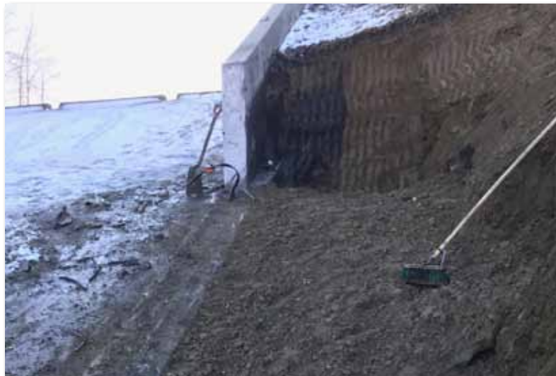
Damaged walls removed and granular backfill placed for proper drainage
