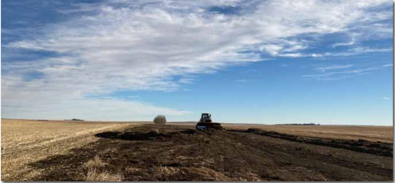
During decommissioning of legacy infrastructure
