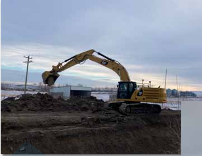
Excavating key trench for liner
