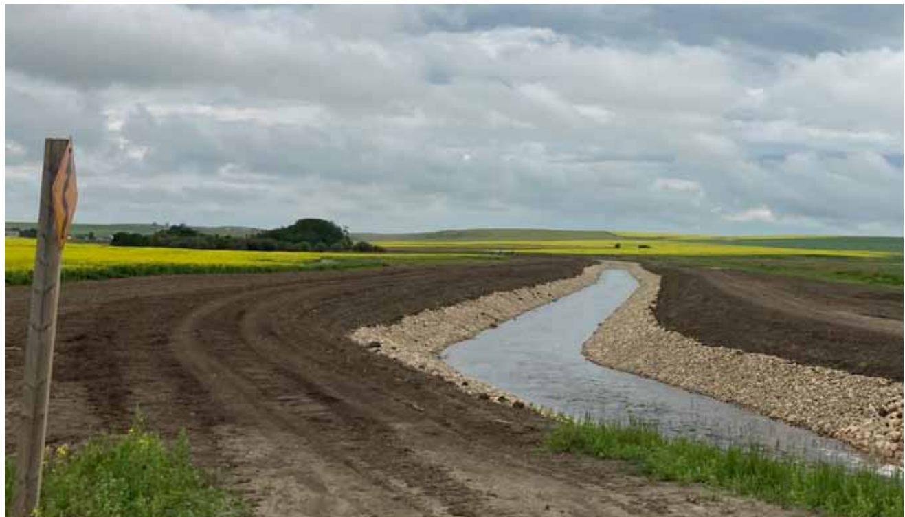
Final phase of North Cluny 3-year IRP Rehabilitation Project is complete
