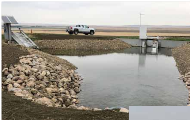
Automated Langemann gate and pipeline screen cleaner
