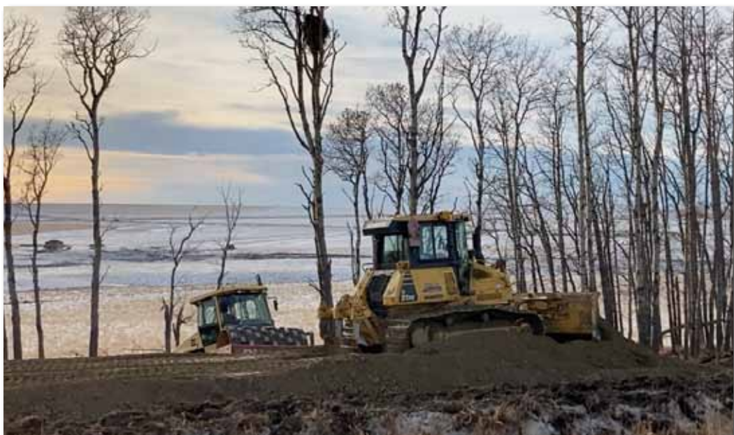
Building and compacting new bank
