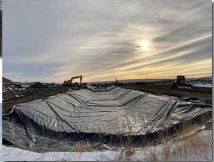
Liner placed in preparation for covering
