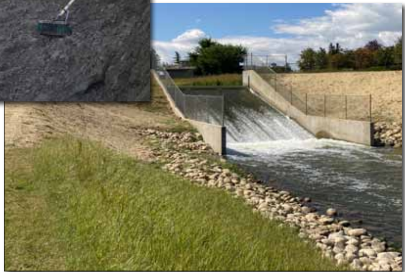
Repaired drop structure operational for 2020 water season
