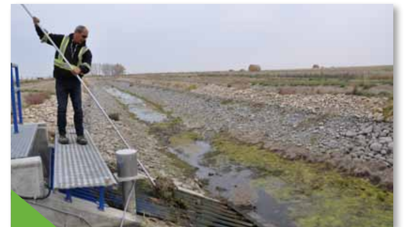
Our Water District Supervisor for Cluny clears weeds and debris from Spillway trash rack
